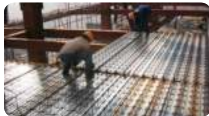
Truss floor board
